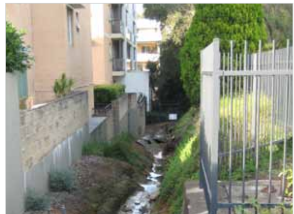
Management and Maintenance: A stormwater flowpath on the eastern edge of the site between the site and the adjacent residential development requires ongoing maintenance providing opportunity to integrate WSUD principles.
