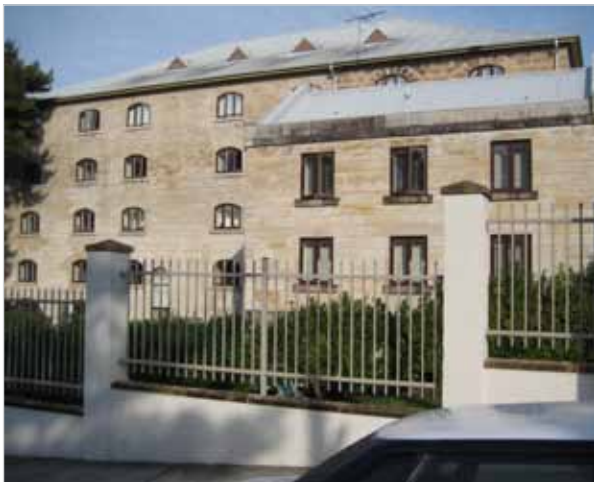
The heritage listed Canterbury Sugar Works (built in 1840) provides an immediate sense of history and place, visually connecting to the Cooks River and the Boat Harbour where sugar cane was shipped from the Philippines.
