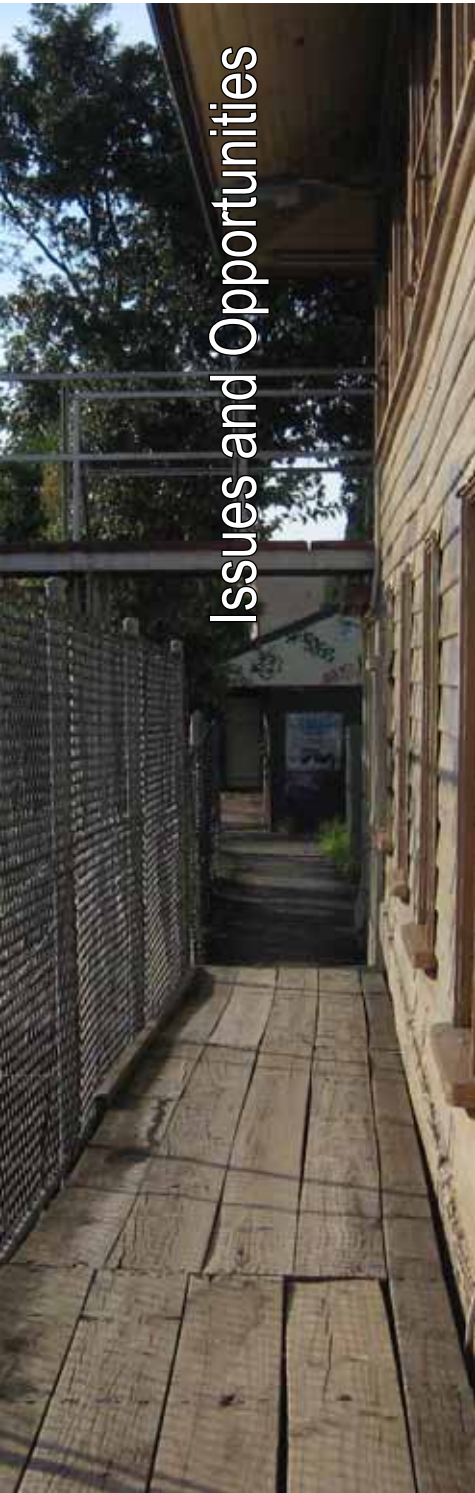
Access between the site and the station is well used by local residents but highly limited by two railway buildings west of the site. This is neither an amenable or safe walking environment.
